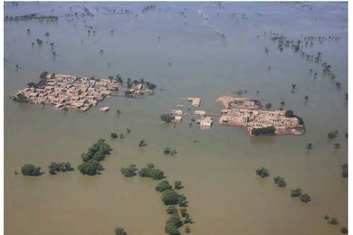
A flooded residential area in the Dadu district of Sindh Province. Husnain Ali/Agence France-Presse — Getty Images
